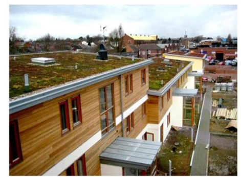
Green roof and roof light in new residential development.
